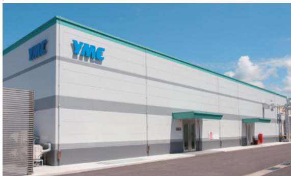
API Purification Plant
